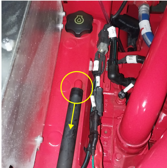
Figure 5. JU4/6 Crankcase Ventilation
